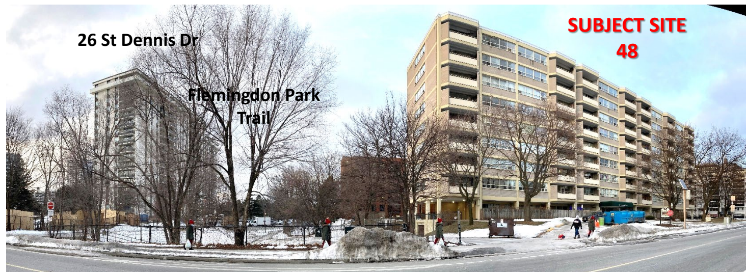
2. View northerly towards 48 Grenoble Drive (Subject Site) and Flemington Park Trail
