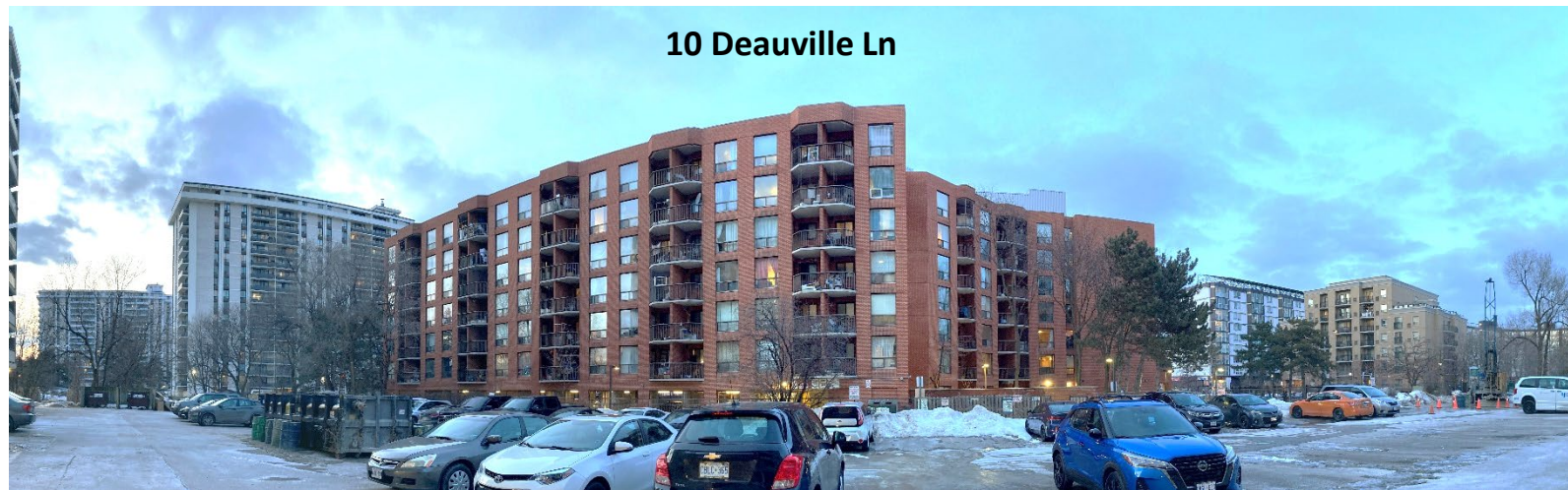
7. View northerly from the rear yard of the Subject Site towards 10 Deauville Lane
